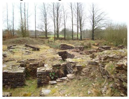
The ruins of the Engine House had been the subject of excavation by The Somerset Industrial Archaeology Society and Exmoor Mines Research Group in the mid/late 1990's. They comprise, inter alia, the remnants of a boiler and engine house (originally with 25 inch beam engine), chimney, water reservoir, balance bob, flywheel pit and gantry piers.
