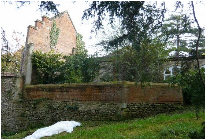
Ruin of original Myrtle Tree Enclosure
