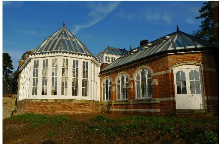
Rebuilt Myrtle Tree Enclosure (left) and Conservatory
