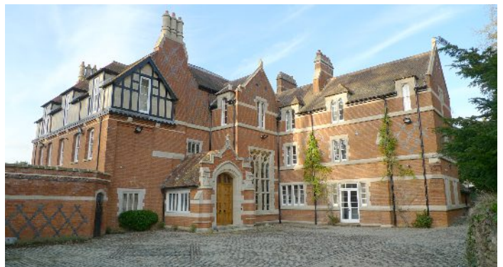
East elevation - newly cobbled courtyard
