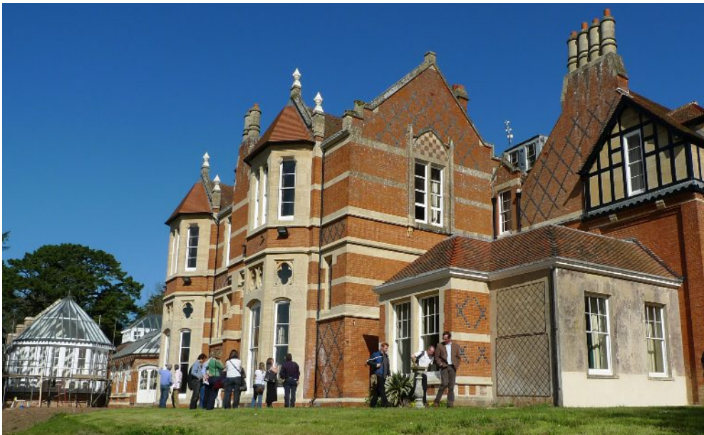
Rebuilt glass houses, finials, hipped bay roofing and restored half-timbered facade
