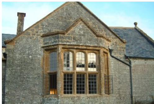
An outstanding example of re-glazing and repair to stone mullion window.
