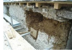
Surface repairs to cob held with oak pegs and deeper repairs to walls.
