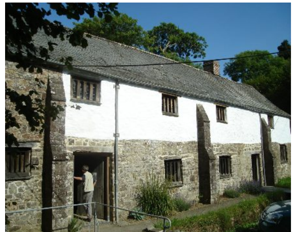
Completed West Elevation.
