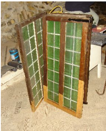
Scarfed timber repairs to windows.
