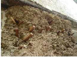
Surface repairs to cob held with oak pegs and deeper repairs to walls.
