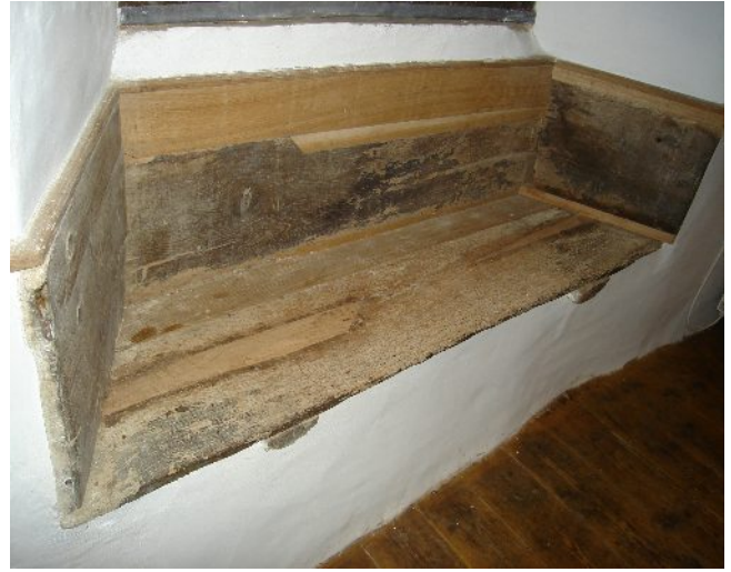
Window seat - repaired.
