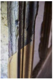
The barn had previously been used to house livestock, and several sections of the internal faces of the salt-rich cob wall had been licked by cows leading to dangerously thin lower wall sections. The walls were carefully propped and trimmed, with new cob repairs to reinstate full structural strength.
